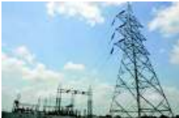
Transmission Line EPC
