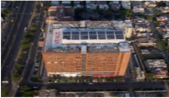
View of Solar Panels on Terrace of Subject Project (provided by Client as Solar Panels on Terrace of Subject Project were not easily accessible)
