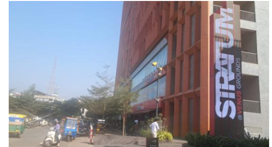
View of Side Access Road to Subject Project
