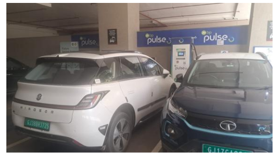
Electric Vehicle Charging Bays at Subject Project
